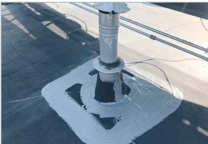
3. Detail penetrations and address ponding areas prior to coating.
